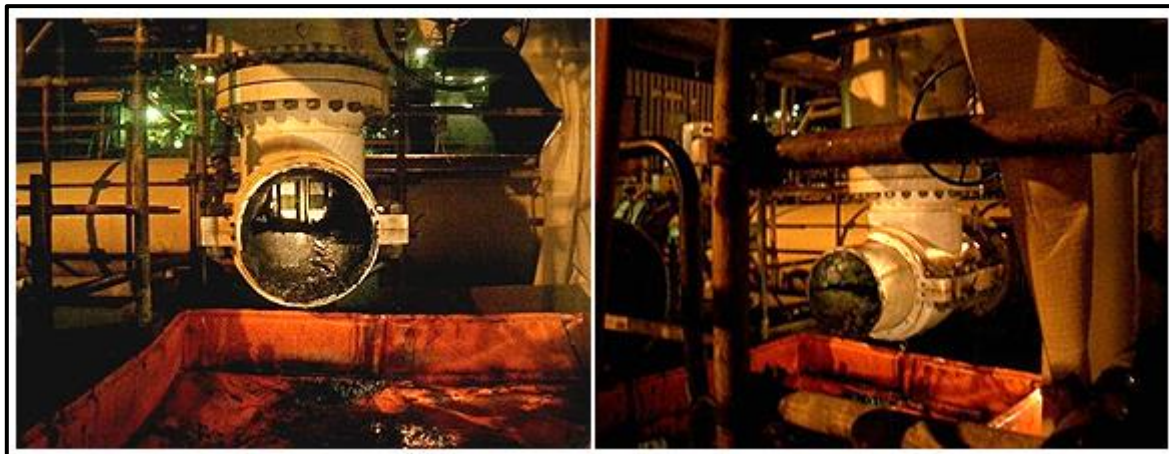
Figure 16. BISEP isolating pipeline on-site with dead leg cut away
