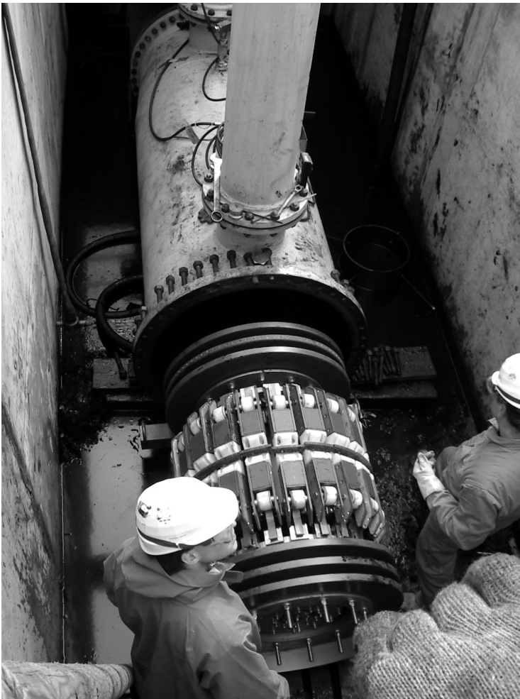
Figure 4: Manoeuvring the Magnetic Flux Leakage Pig into the Pipeline
