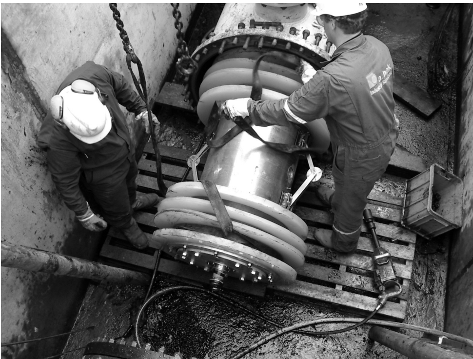
Figure 3: Manoeuvring the Ultrasonic Pig into the Pipeline
